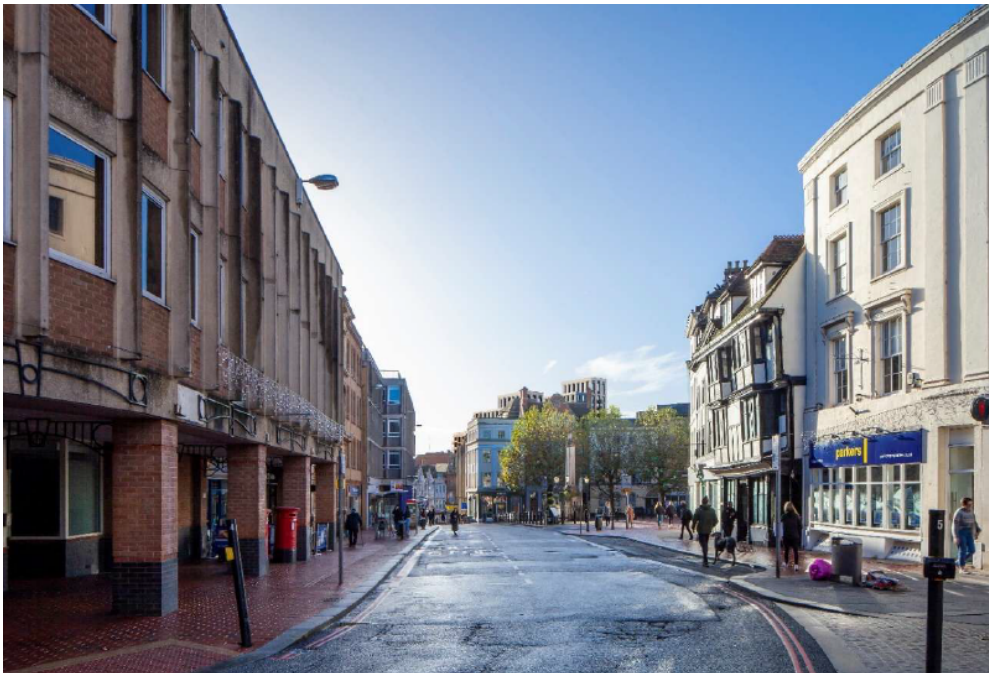
Figure B – Proposed view of the YHP2 development looking south from Market Place from the junction with The Forbury
